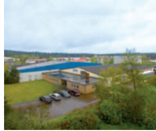
Plant Mölln (Germany)
